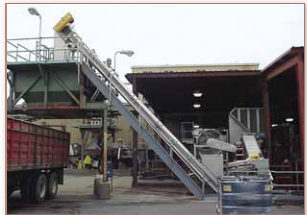
Installation of 24SWR.
